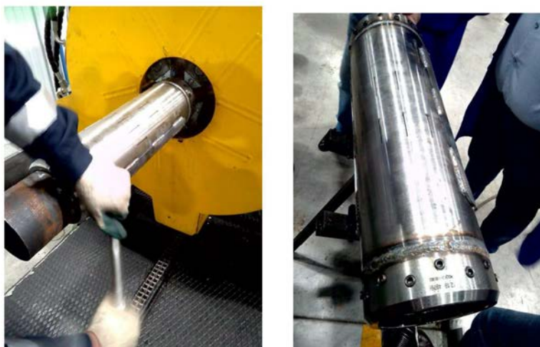
Figure 5—Marker cassette prototype model installation on a base pipe.
